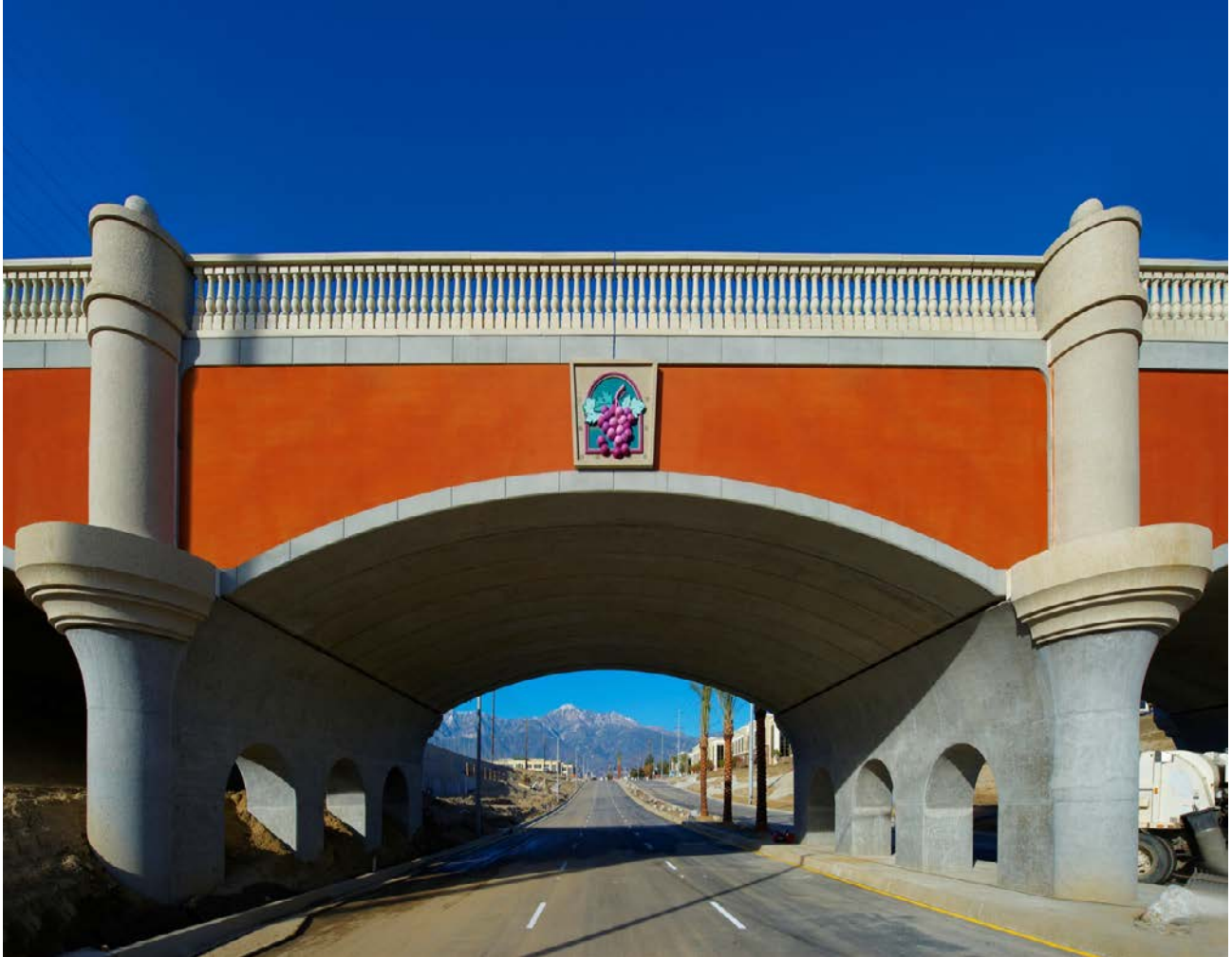
Metrolink trains now pass over the Haven Avenue Grade Separation in Rancho Cucamonga, which is just one of many new grade separation projects in SANBAG's service area.
