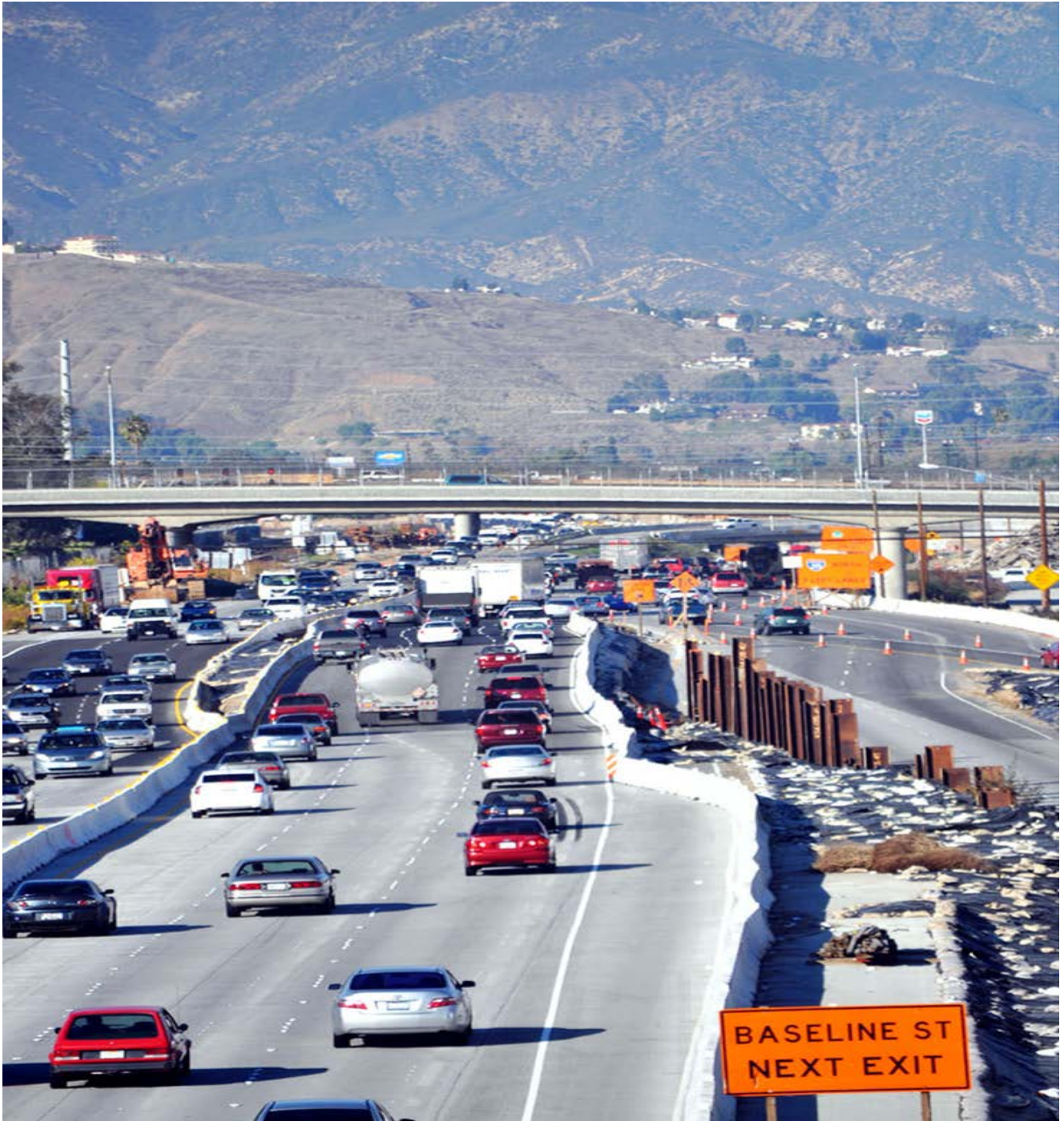
Reconstruction of the I-215 Freeway through San Bernardino spanned over seven years, from 2007-2013, at a cost of $723 million.
