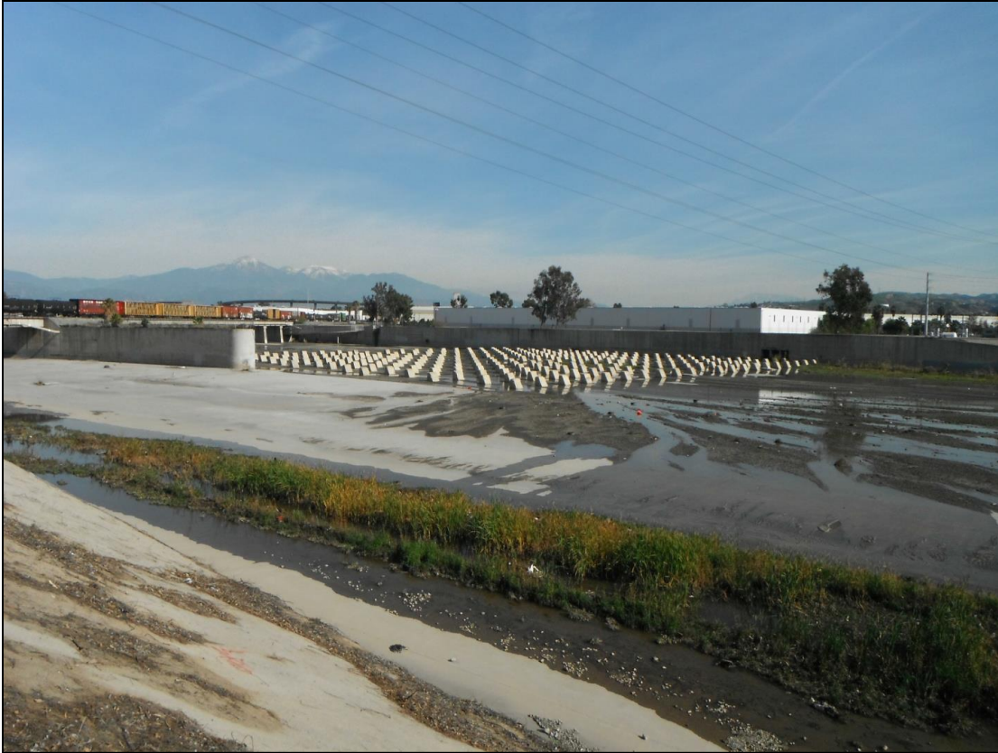
Figure 3.3.5-2 Santa Ana River Channel – South of I-10 Facing Northeast
