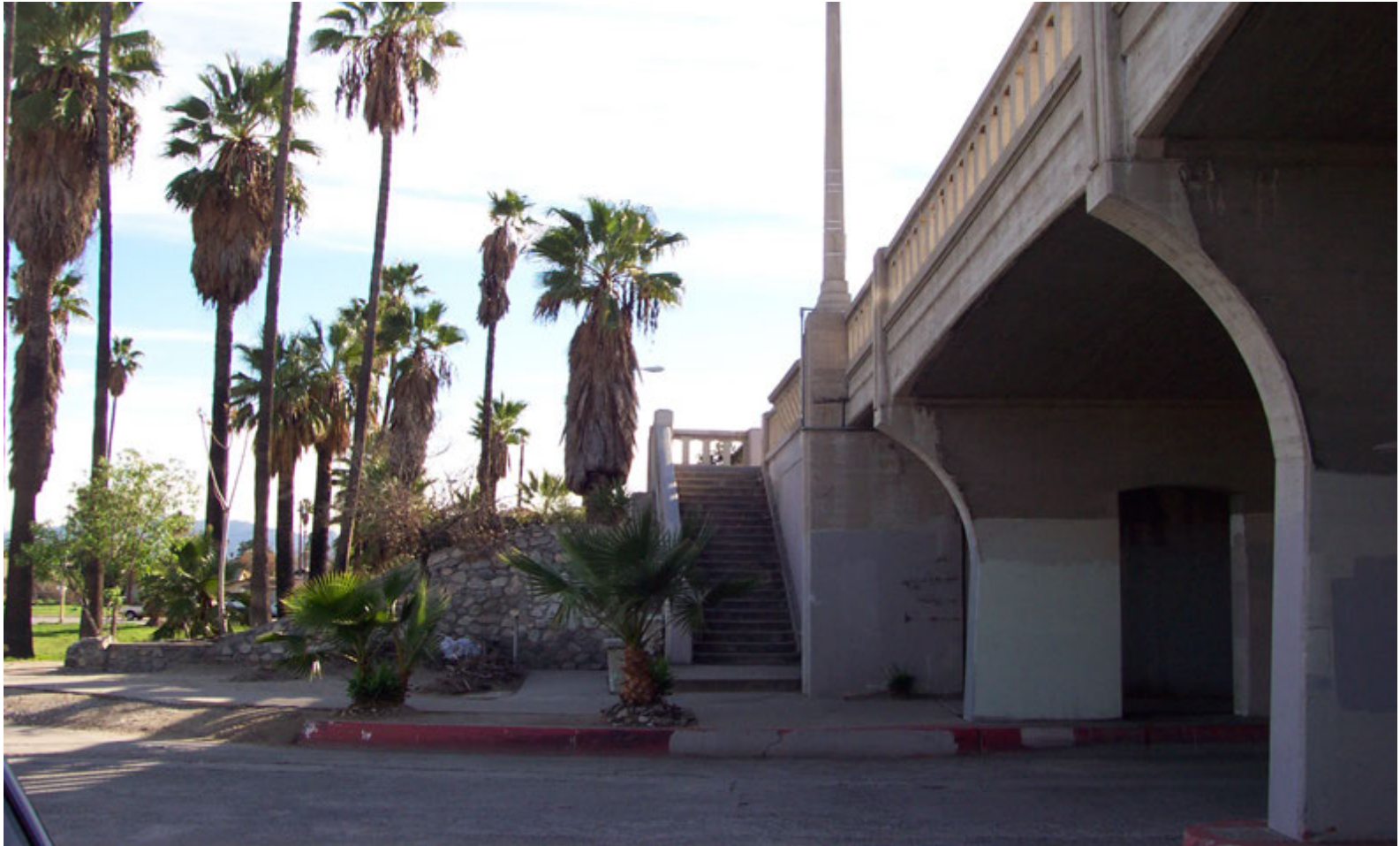
Looking south along the east side of the bridge, January 15, 2004. At the center of the image is the stairwell at the southeast corner of the bridge, a character-defining feature. To the far right are Abutment 1, and Bent 2 and 3, all character-defining features.
