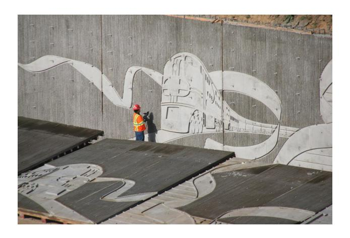
Crews from the Interstate 215 Bi-County HOV Project work on the newly formed aesthetic retaining walls between Interstate 10 and State Route 60.
