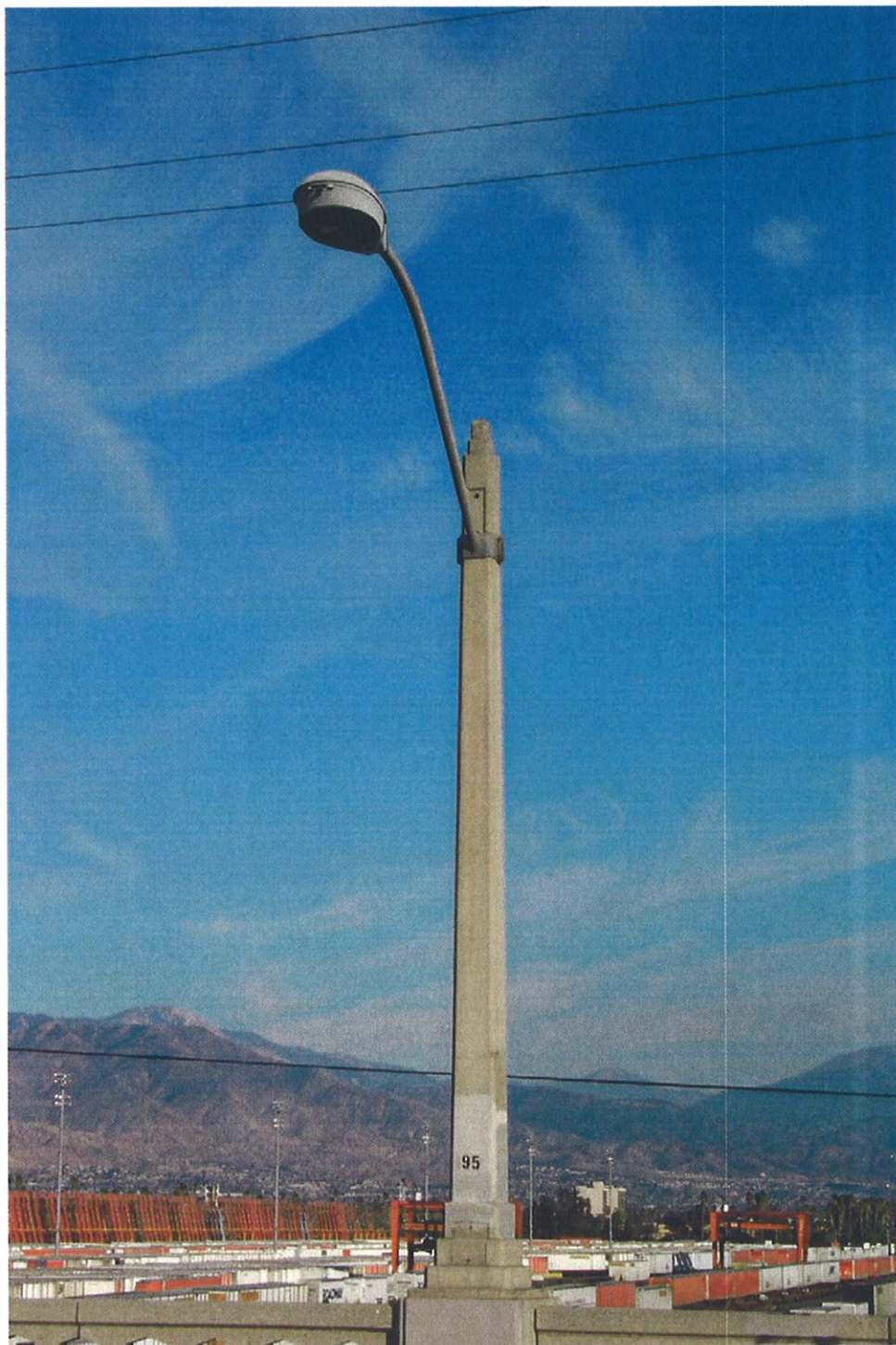
An example of an original light pole, with a modern “cobra” lamp, January 15, 2004. The pole is part of a character-defining feature.
