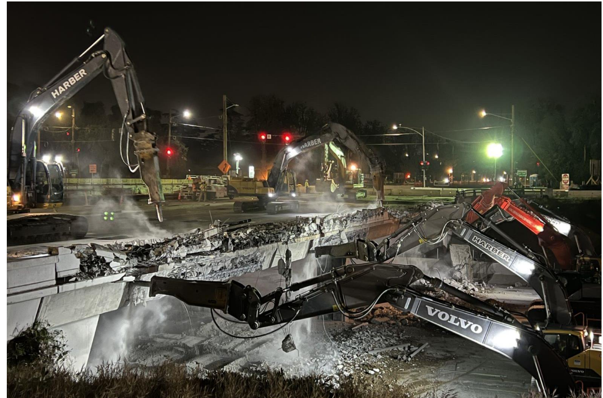
Partial demolition of Euclid Avenue Bridge on I-10 Express Lanes Project
