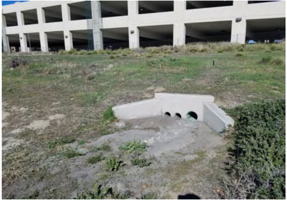
Photograph 9: View of stormwater drainage pipe that discharges to vacant land. Stormwater is likely collected from nearby parking structures.
