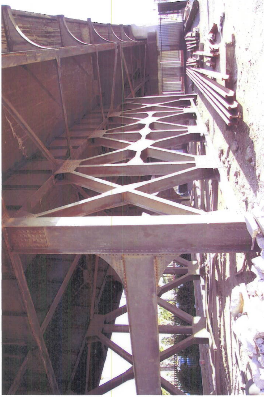
Looking northwest at the steel arched brackets, which support the bridge deck and are character-defining features. Image taken on January 15, 2004.
