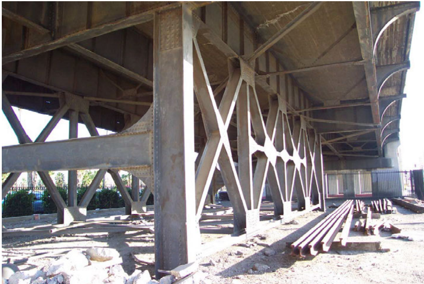
Looking northwest at the steel arched brackets, which support the bridge deck and are character-defining features. Image taken on January 15, 2004.
