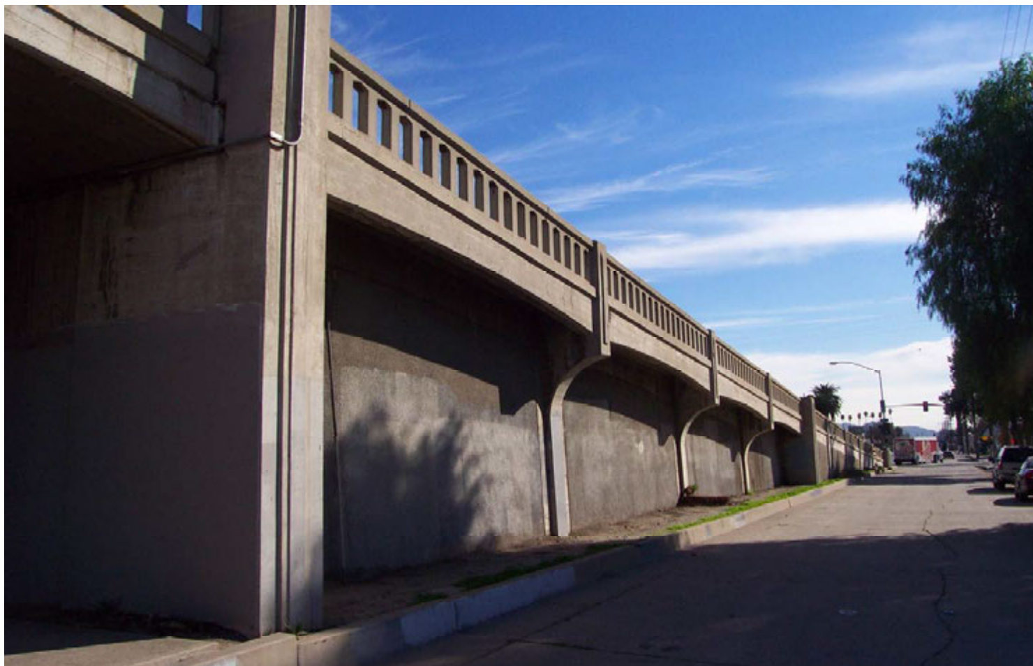
This image was taken looking south/southeast along North Mount Vernon Ave, January 15, 2004. It shows some of the bridge railing and the over hanging sidewalk deck, which are both character-defining features.
