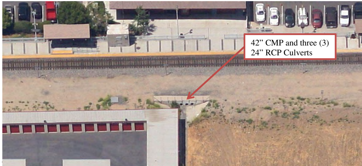
Figure 3-11. Drainage Culverts at the Rialto Station – Looking North
