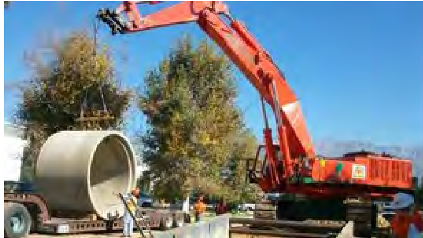
Figure 3-19. 120” Storm Drain Installation at Hellman Avenue
