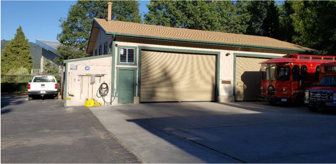
Figure 5-6. Crestline Base's Maintenance Facility
