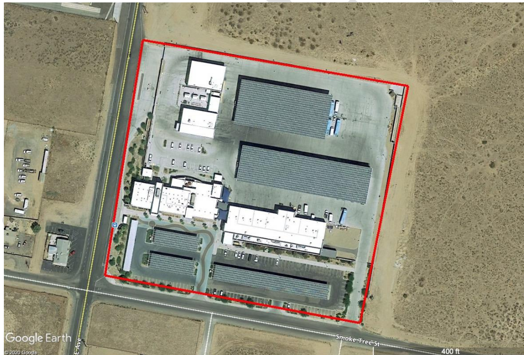
Figure 8-4. Hesperia Yard - Existing Conditions
