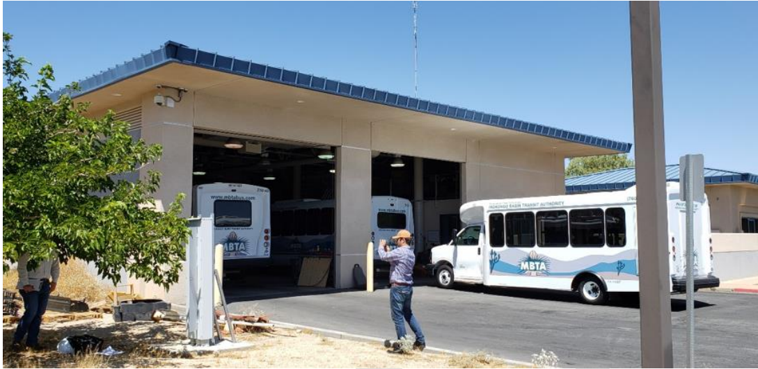
Figure 4-5. Joshua Tree Yard's Maintenance Facility
