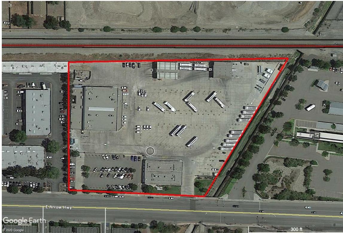
Figure 7-6. West Valley Division - Existing Conditions
