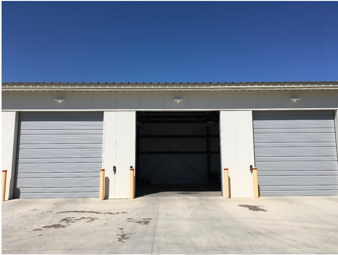
Figure 6-4. NAT Garage - Existing Conditions
