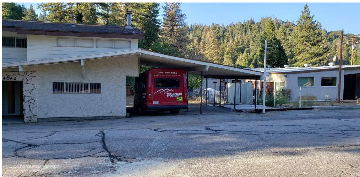
Figure 5-14. Crestline Base (Future) - Existing Conditions
