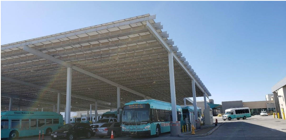
Figure 8-6. Hesperia Yard's ChargePoint Chargers and BEBs
