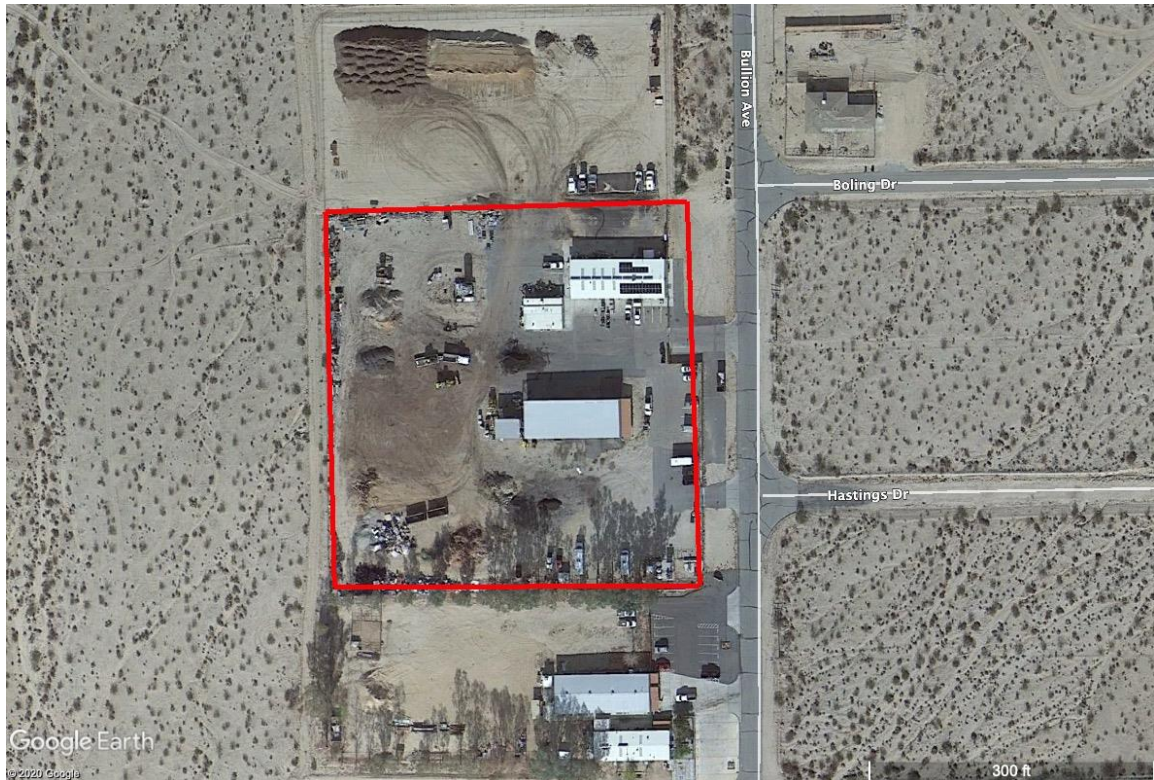
Figure 4-7. Twentynine Palms Yard - Existing Conditions
