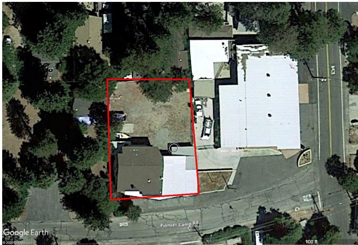
Figure 5-13. Crestline Base (Future) - Existing Conditions
