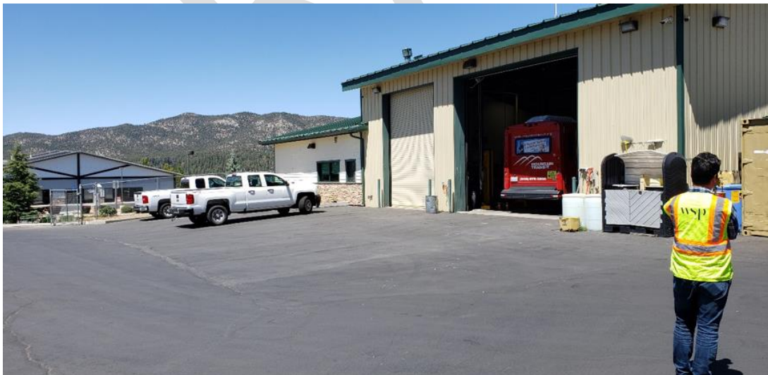
Figure 5-10. Big Bear Lake Base's Maintenance Facility
