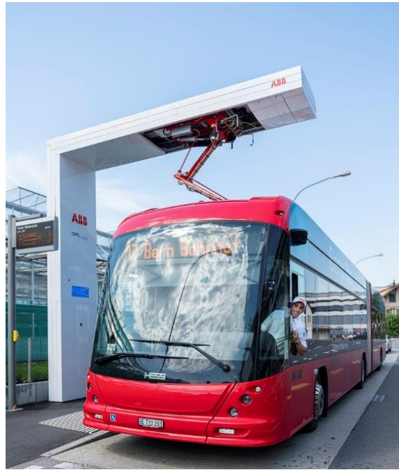
Figure 1-15: ABB Designed On-Route Charger in Bern, Switzerland
