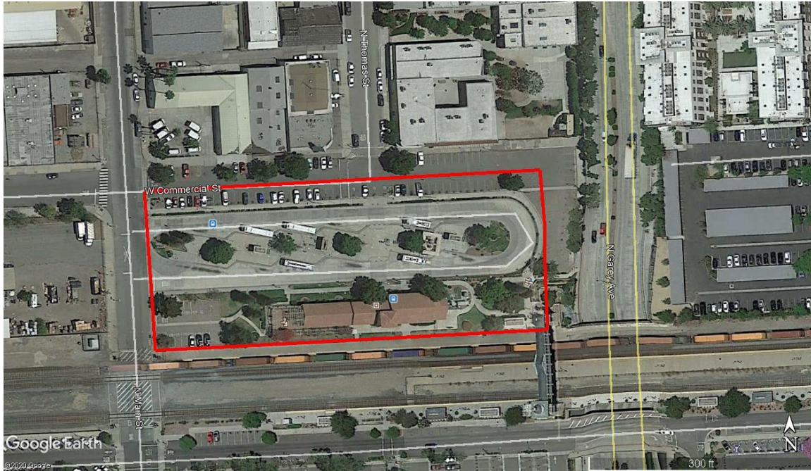
Figure 6-19: Pomona Transit Center – Existing Condition
