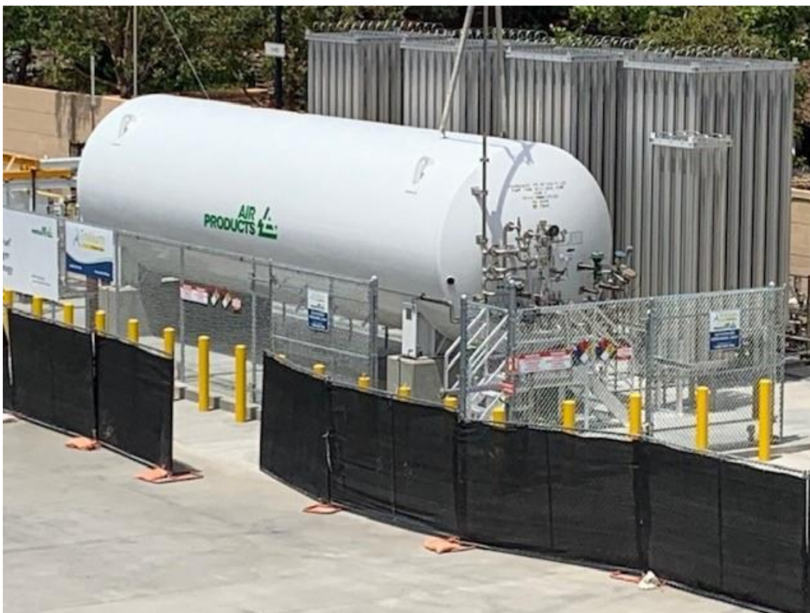
Figure 1-23: OCTA's 4,500 kg Hydrogen Tank
