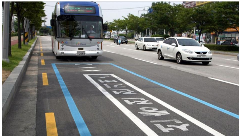
Figure 1-22: Gumi's Inductive Charging Lane
