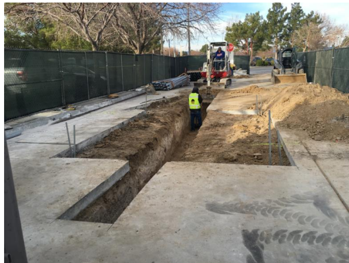
Figure 1-19: Construction of AVTA's WAVE Charger
