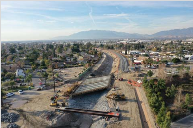
Mountain View Track Construction & IVDA Bridge work – January 2021
