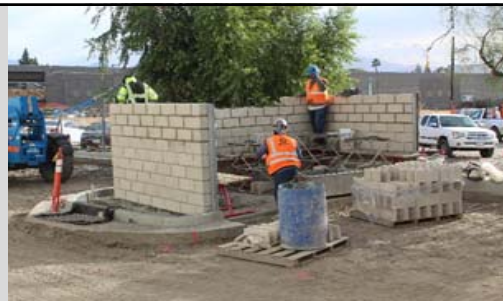
CMU trash enclosure constructed
