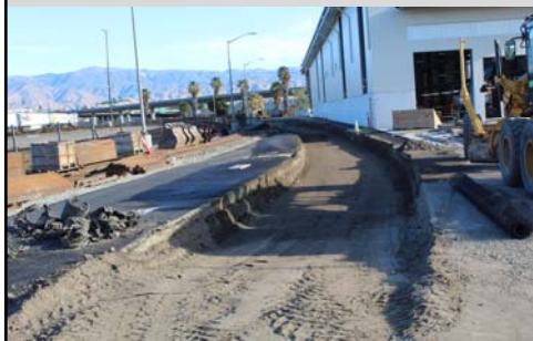
Yard Track Excavation
