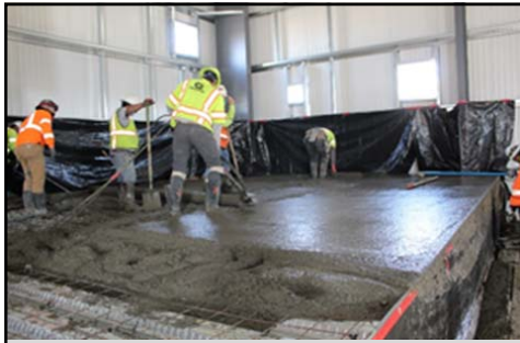
Mezzanine deck placement
