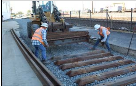
Laying out ties for Yard Track 1
