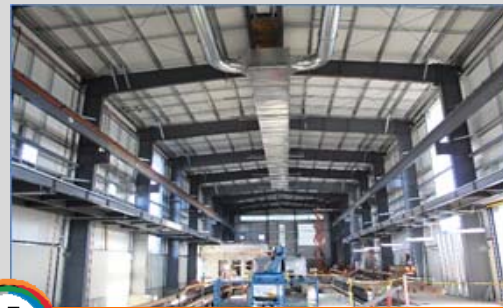
HVAC installation continues
