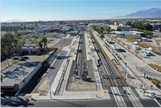
SBTC Station – January 2021
