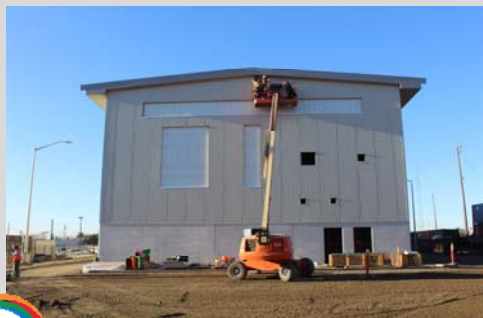
Installation of exterior translucent panels
