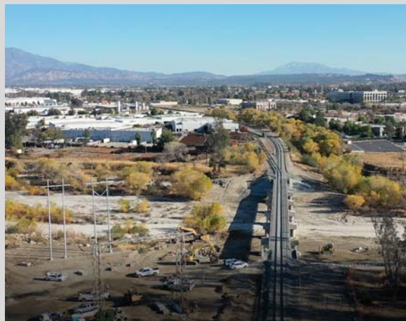
Santa Ana River Bridge - January 2021
