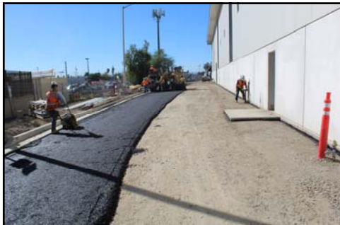
AC base course placed for entire site
