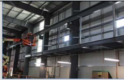
Fall protection post installation
