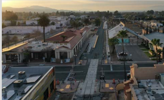
Downtown Redlands DMU & SCRRRA Platforms – January 2021
