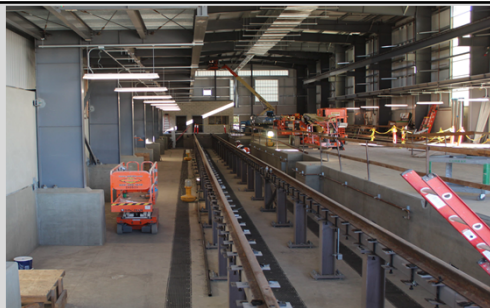
Posted Rail Pit
