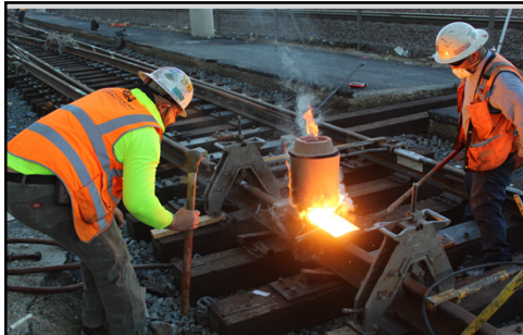
Constructing yard track
