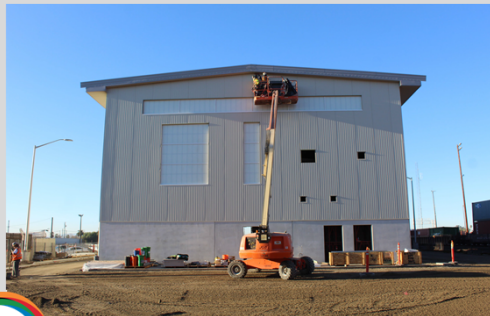
Installation of exterior translucent panels
