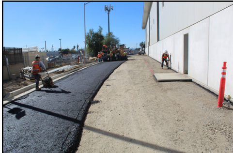
AC base course placed for entire site
