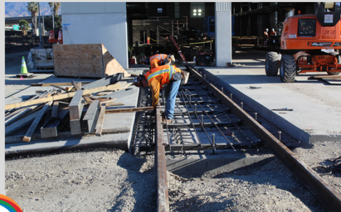
Constructing Yard Track 4 at approach apron
