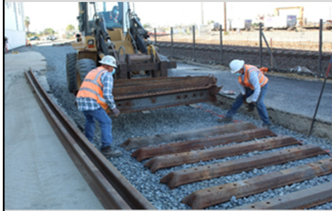
Laying out ties for Yard Track 1
