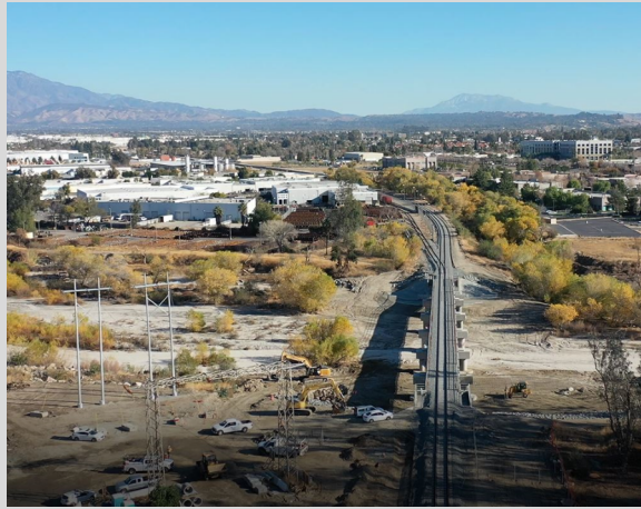
Santa Ana River Bridge - January 2021
