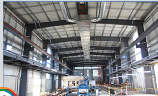
HVAC installation continues
