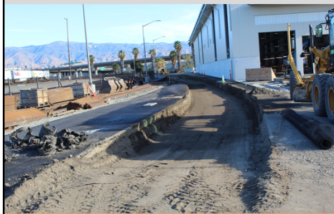
Yard Track Excavation
