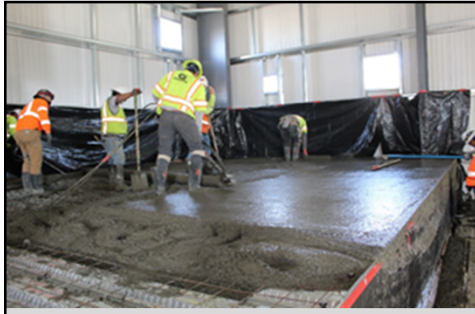
Mezzanine deck placement
