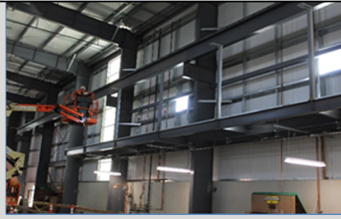
Fall protection post installation
