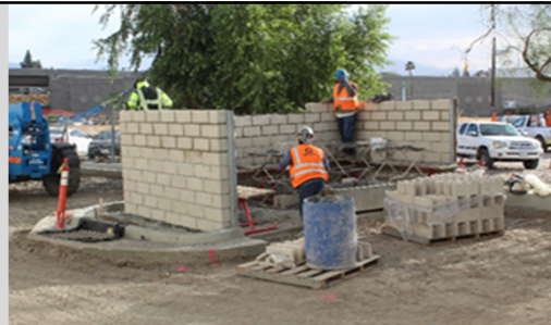
CMU trash enclosure constructed
