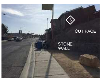
PHOTO 2831 FOUNDATION 3 (RESIDENCE) NO SCALE
