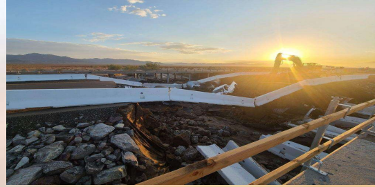
I-10 Washout (Diversion Lane)
