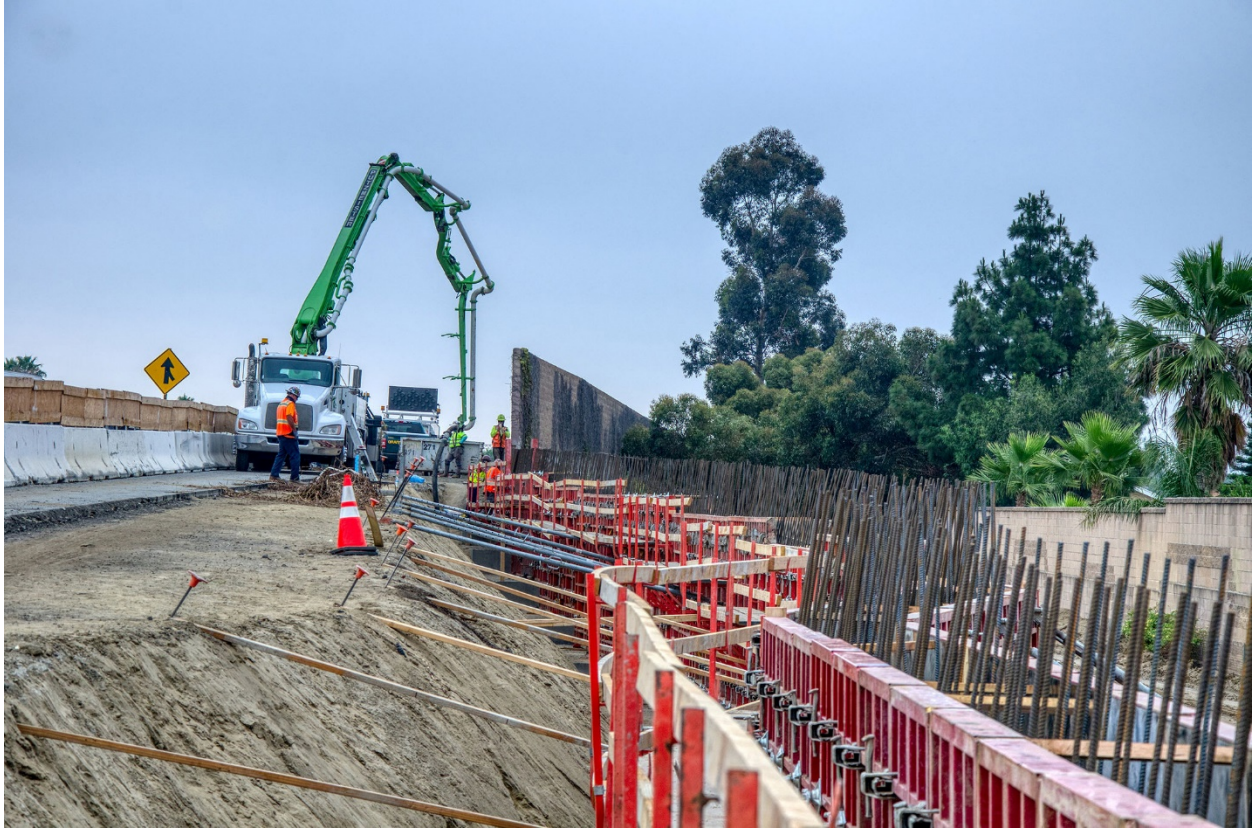
Widening the ramps at Archibald Avenue along State Route 60 in Ontario is no small task. Crews are shown here setting the foundation for retaining and sound walls along the new outer edge of the ramps.
