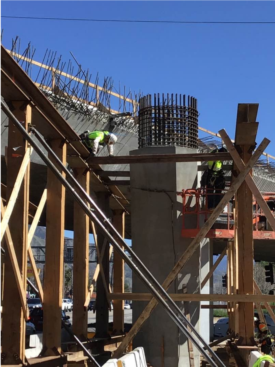
State Route 210 is a major connection to the east valley of San Bernardino County, as well as the San Bernardino Mountain Resorts. Crews are shown here setting the “falsework” or temporary support system for the reconstruction of one of the many bridges being widened to accommodate the additional lane in each direction.
