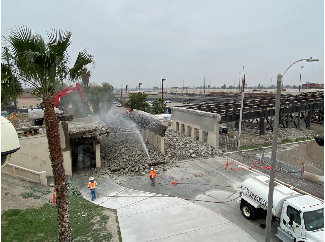
Crews begin the strategic disassembly of the old Mount Vernon Avenue Viaduct over the Burlington Northern Santa Fe Railroad (BNSF) rail yard in San Bernardino. This structure is nearly a century old and serves as a key connector to one of the older communities in San Bernardino.
