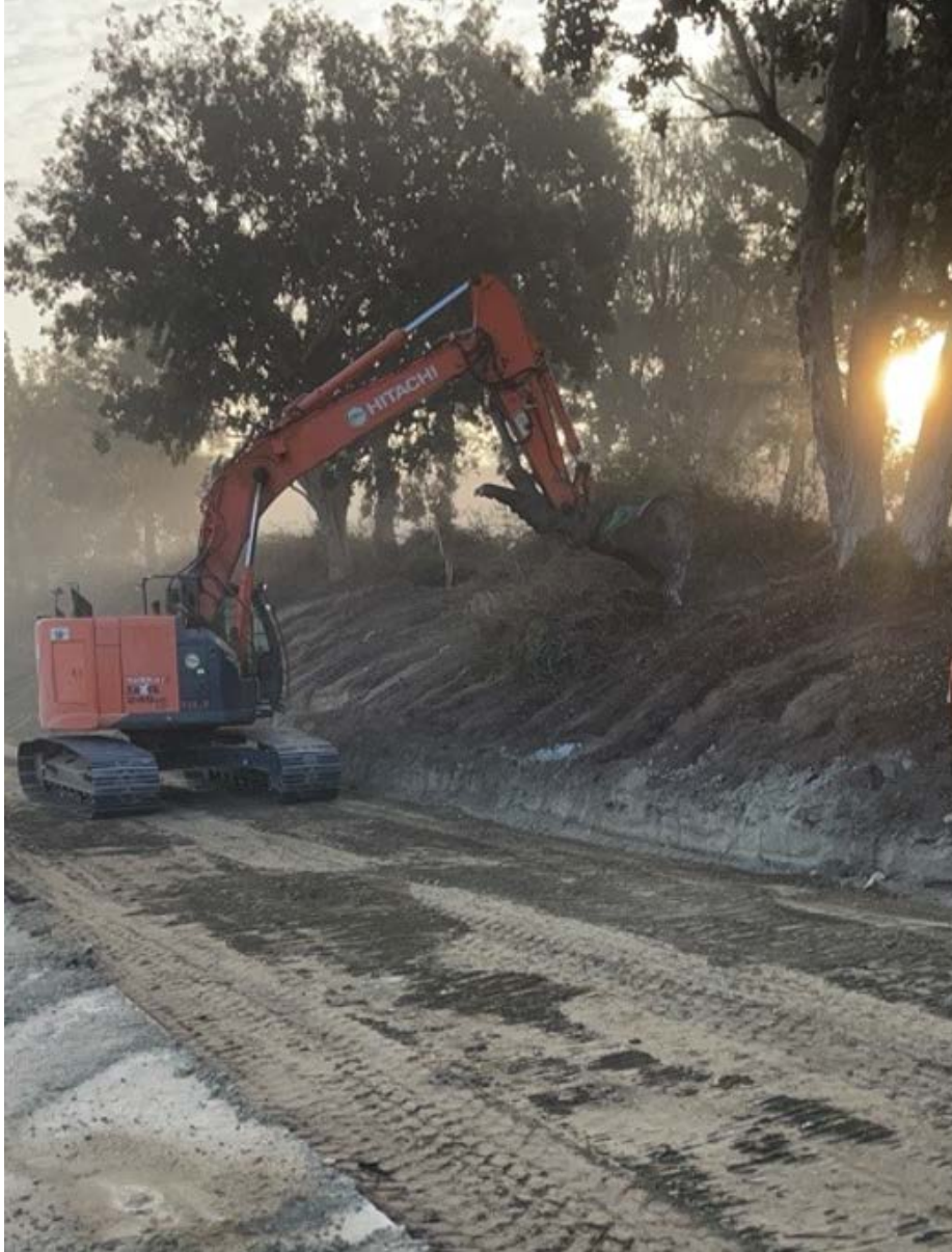
Early morning crews excavate a slope to allow for the widening of ramps at State Route 60 and Central Avenue in Chino.
