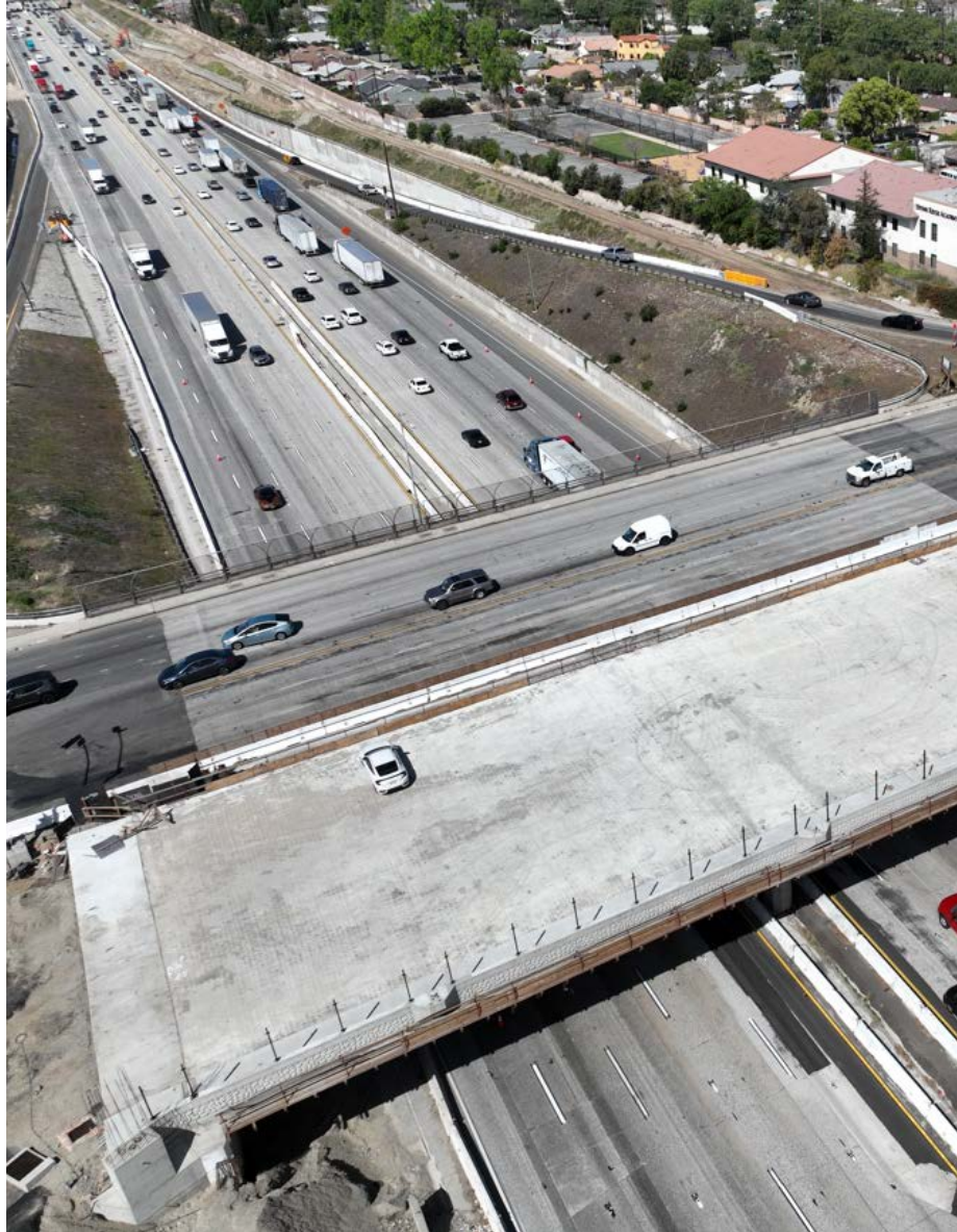
Euclid Avenue under reconstruction as part of the Interstate 10 Express Lanes Project. This major interchange was built in two phases to allow traffic to continue during construction.
