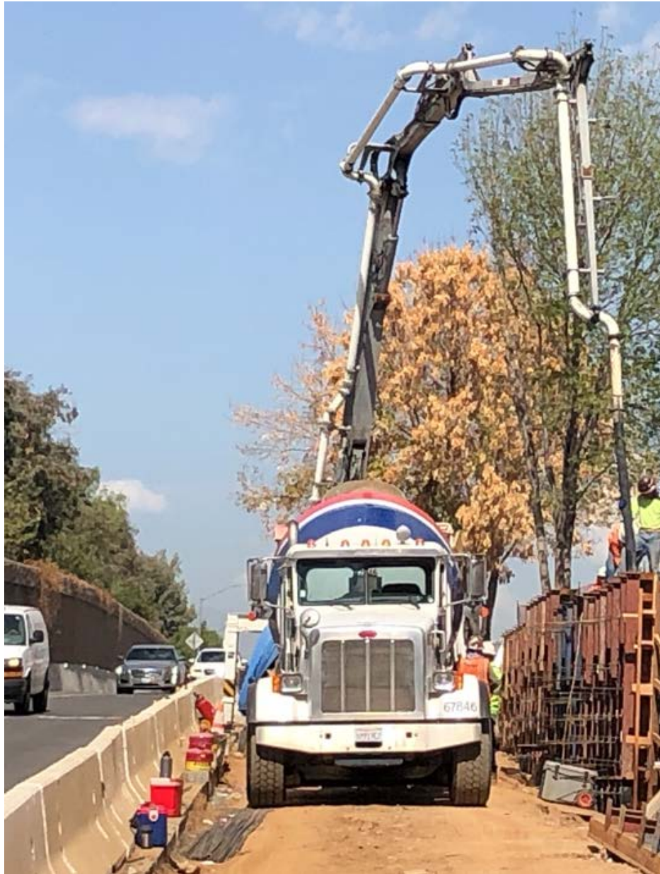
A pumper trucks supplies the concrete used in the footings for new retaining walls at the Interstate 10 University Interchange in Redlands.
