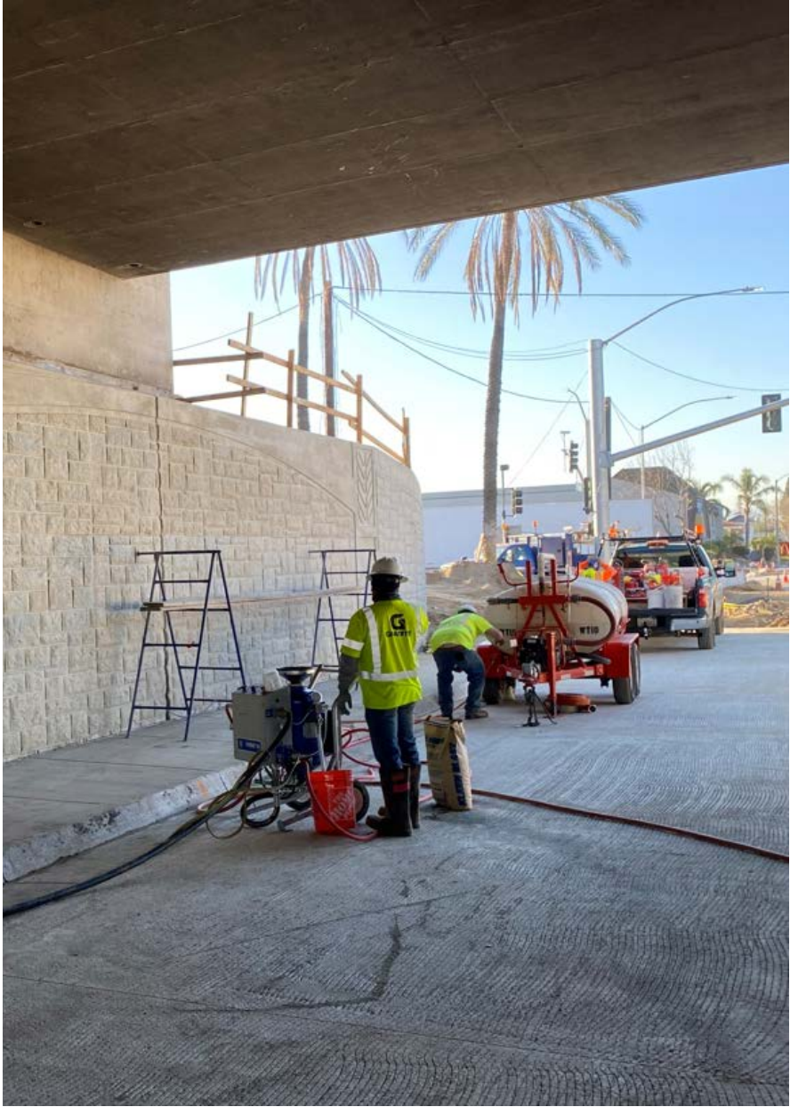
Applying context sensitive solutions is an important part of projects in the various communities throughout the county. Wall aesthetics are just one way to celebrate history and culture.
