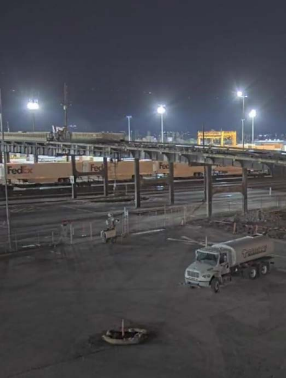
Nighttime crews prepare for the daytime demolition of the old Mt. Vernon Avenue Bridge in San Bernardino. This iconic structure is being replaced after nearly a century of service to the community.
