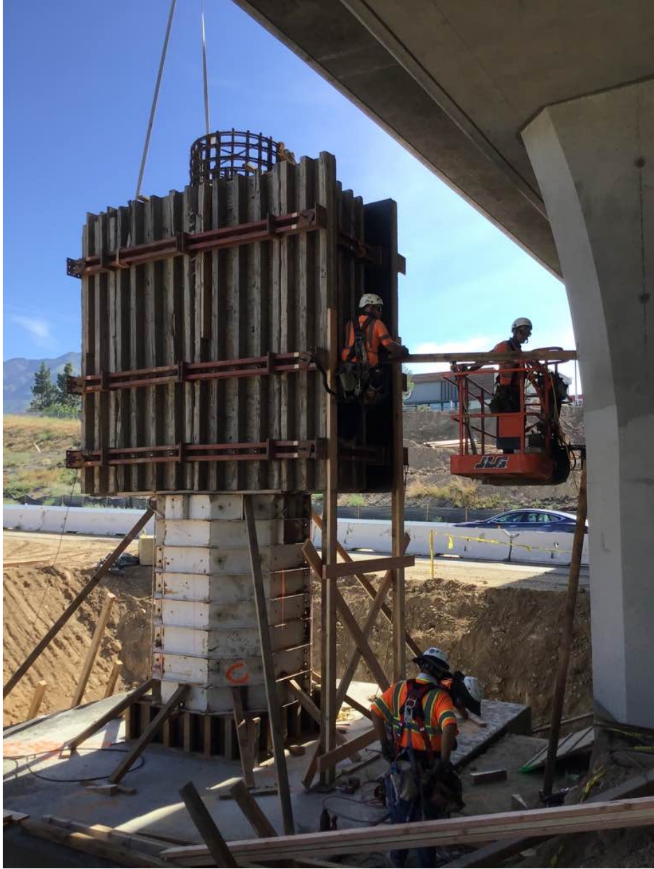
Large wooden forms are built to construct bridge columns at the Baseline Interchange on State Route 210 (SR 210) in Highland.
