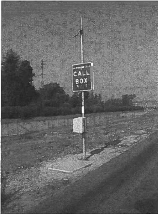
Site Type A – installed at-grade, in soil.
