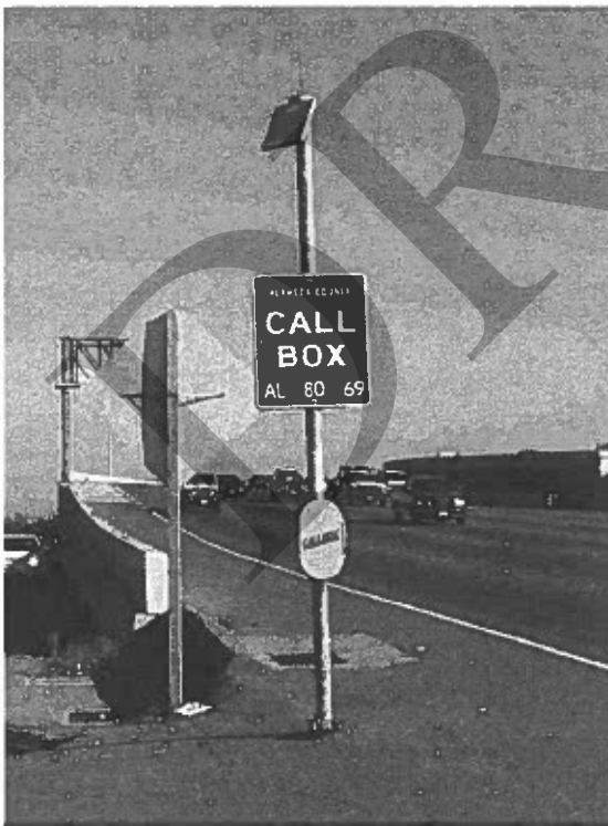
Site Type G – installed at-grade, in concrete.
