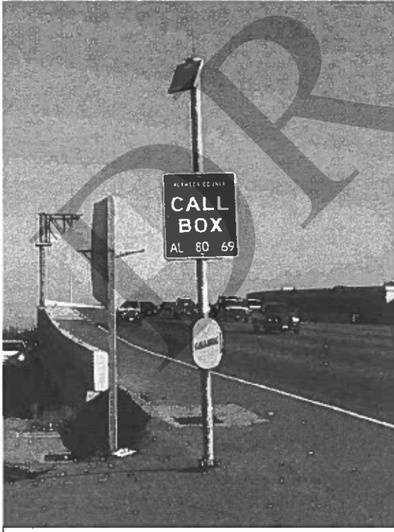
Site Type G – installed at-grade, in concrete.
