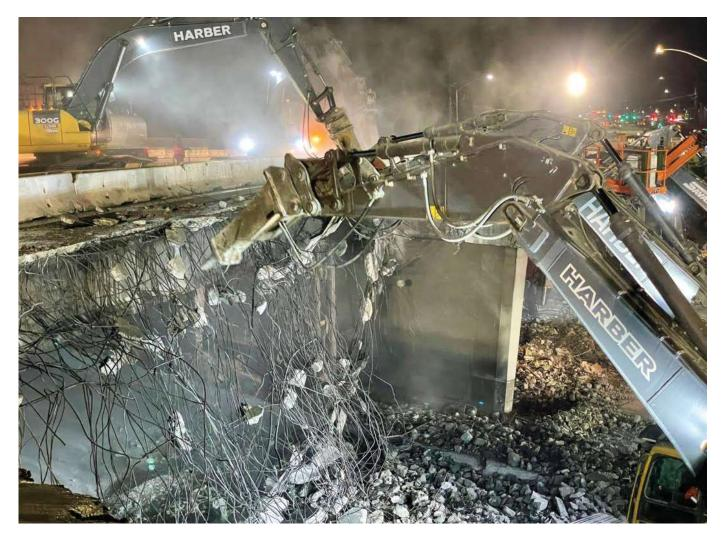
Under the bright lights brought in for crews to work safely at night, the project team is busy demolishing a bridge over Interstate 10 in preparation for the future Express Lanes. Work like this is often done at night because it requires the lanes below to be closed for safety. Closing during the day would impact hundreds of thousands of commuters.
