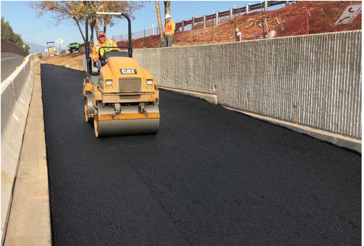
Crews drive heavy rollers over freshly placed hot mix asphalt to serve as the foundation for new ramps on Interstate 10 in Redlands.
