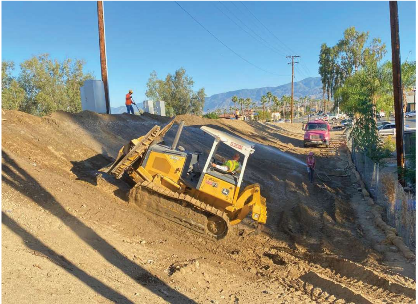
SBCTA is phasing in improvements to various ramps throughout the county. Crews are grading the slopes of part of the widened ramp access to and from Alabama Street in Redlands.
