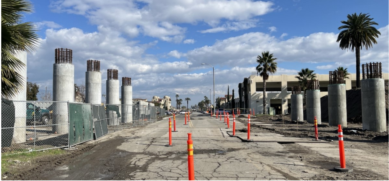
New columns rising out of the ground in preparation of the new bridge spanning over the Burlington Northern Santa Fe Railroad (BNSF) rail yard in San Bernardino.
