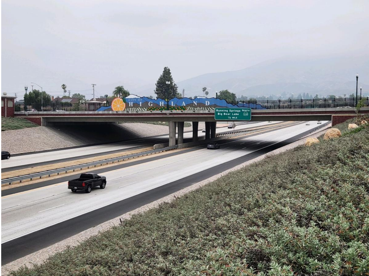
The City of Highland adorned the new bridge at Baseline at State Route 210 with a sign showcasing its pride as the gate way to the mountain communities. The bridge was reconstructed as part of the State Route 210 Lane Addition Project.
