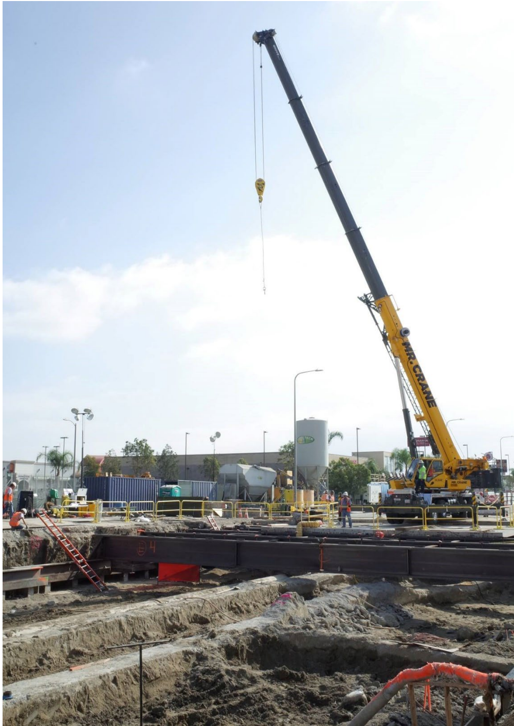
Figure 1: Example of Construction via Cut-and-Cover
