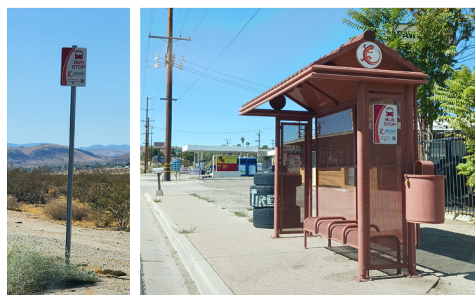
Figure 57: Bus stop examples - On the left, a stop with minimal presence, and on the right, a sheltered stop with seating, trash receptacle, lighting, signage, sidewalk and curb separation from the road. Ideally, all improved high priority stops would reach this level of amenities.
