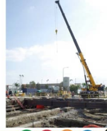
Example of Cut-and-Cover Construction
