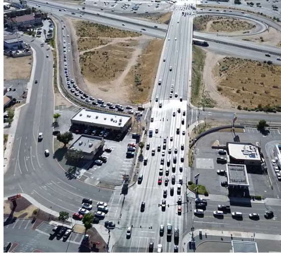
Aerial of the I-15 interchange at Bear Valley Road
