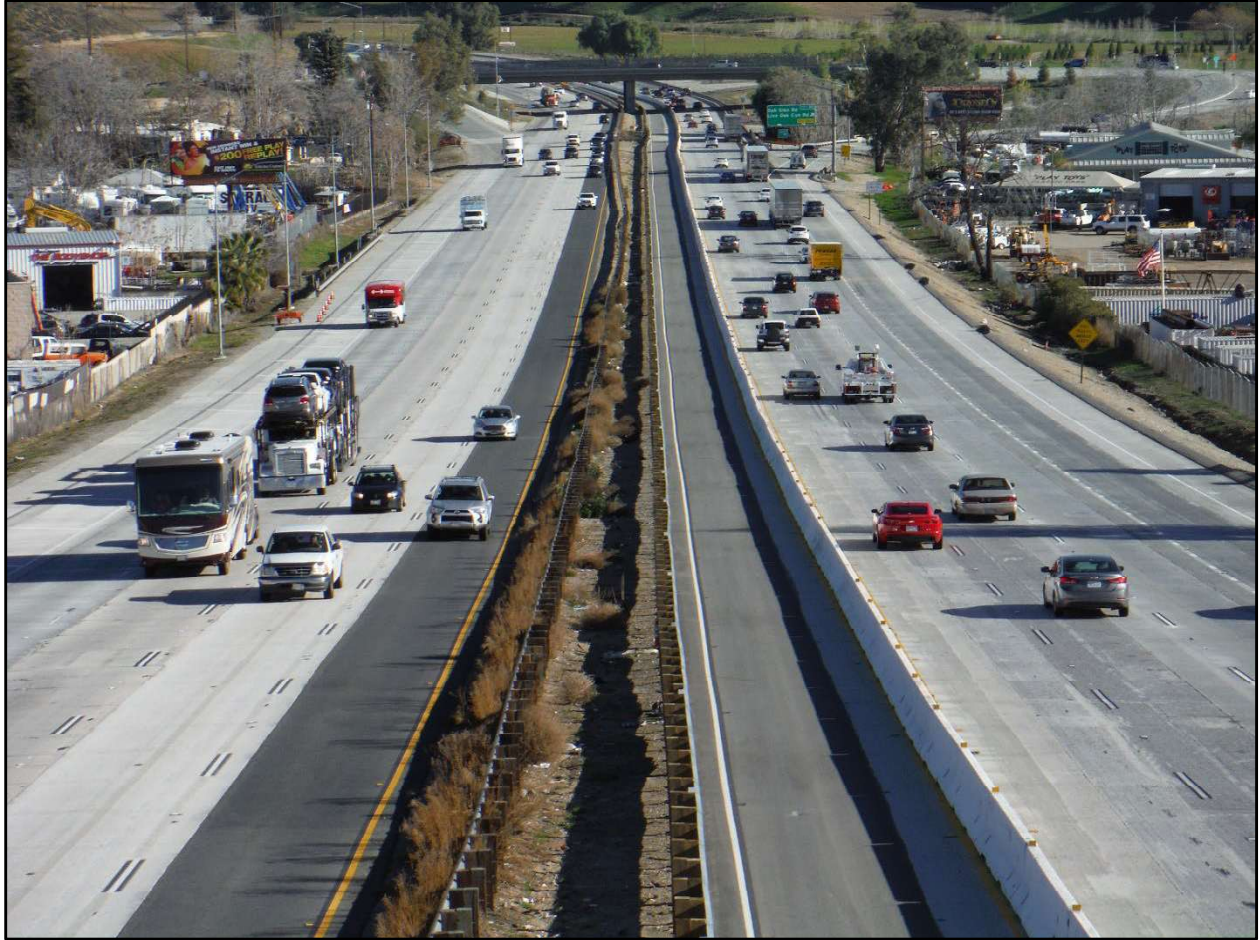
Interstate 10 (I-10) Truck Climbing Lane: A wide view of the I-10 freeway showing multiple lanes of traffic moving in both directions, with a newly constructed truck climbing lane and upgraded pavement.
